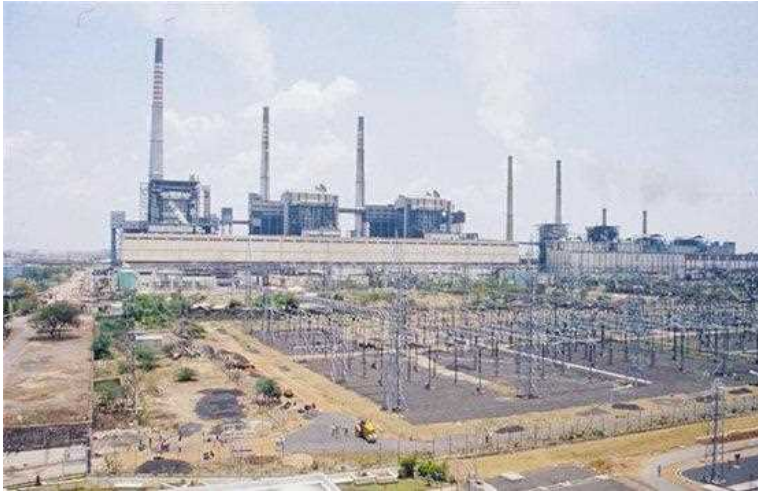
Chandrapur Power Plant
