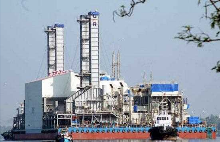
Kakinada Power Plant
