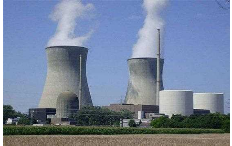
Kakarapar Atomic Power Station Project, Gujarat
