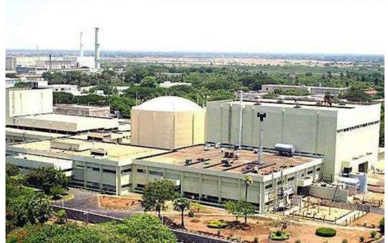
Kalapakkam Atomic Power Station
